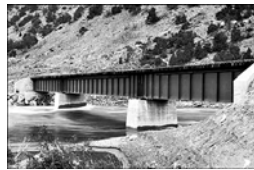
(A) Beam bridge, aspect ratio \approx 10
