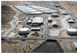
Fort Irwin Water Plant nears completion
